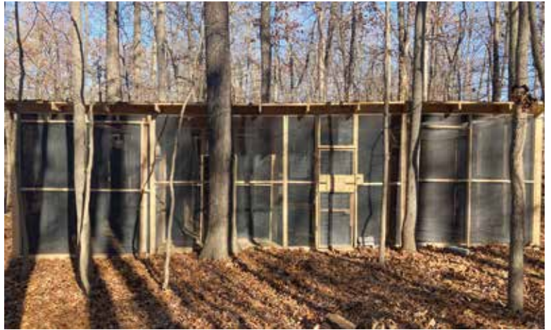
Refurbished songbird complex built by Boy Scout Troop 961.
